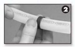
Step 2. Slide the correct size crimp ring over the tubing and approximately 2" past the end of the tubing.
