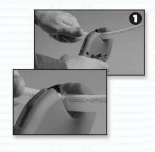
Step 1. Use plastic tubing cutters to cut the tubing between the pointed ends of the repeating 1" SharkBite® imprint pattern. The pattern provides a visual aid to determine if the tube has been inserted all the way into the fitting. Ensure the tube is cut square. A square cut end allows the tubing to be inserted all the way into the fitting. Ensure the tube has no rough edges, cuts or abrasions (rough edges, cuts or abrasions may damage the O-ring and cause the fitting to leak).
