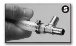
Step 5. Verify the connection is secure by visually checking the clamp tab.
